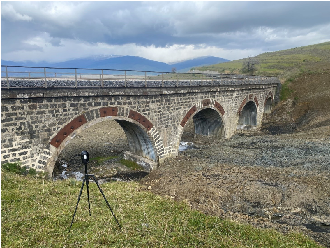
Figure 25 - The Maletto bridge during the 2022 survey campaign
