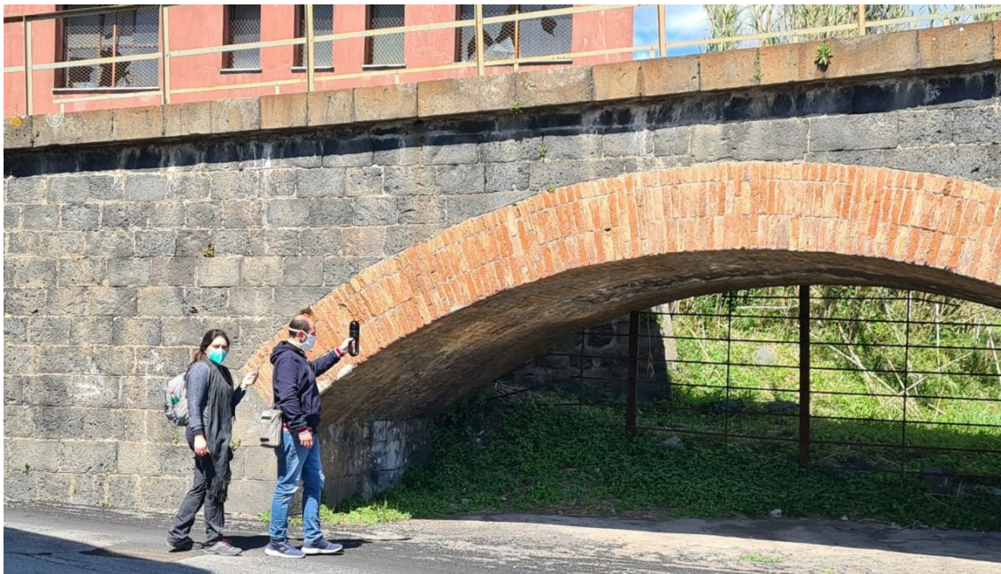
Figure 18 The bridge survey using the BGLK2GO
