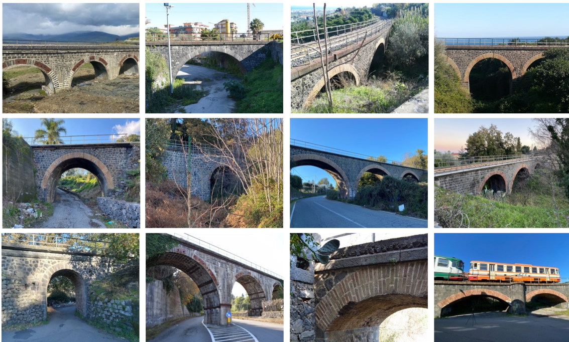
Figure 6 – Top: Identification of bridges along the Riposto-Castiglione section; bottom: some of the masonry bridge along the Circumetnea rail line
