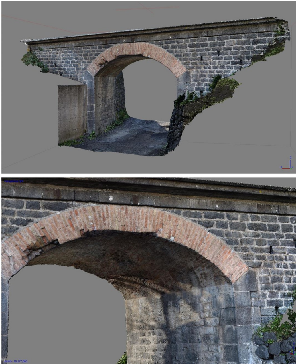
Figure 22 The dense point cloud reconstruction of the bridge
