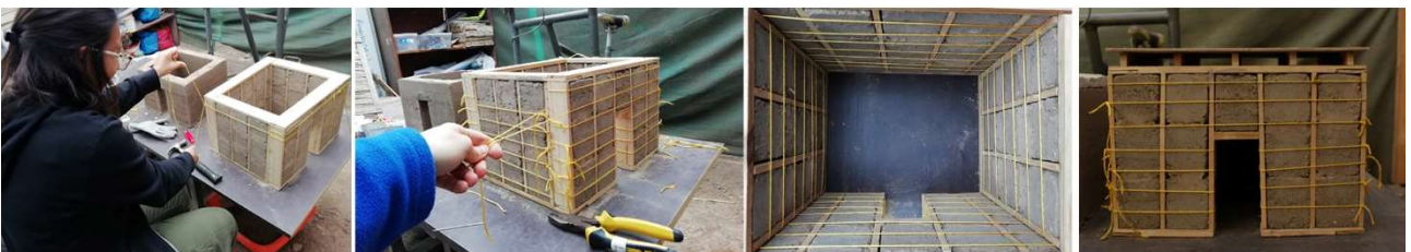
Figure 26 – Some construction phases of the tree scaled prototypes.
