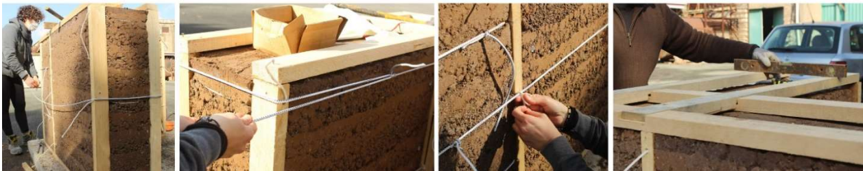
Figure 37 – Full scale prototype construction phases (F-I).
