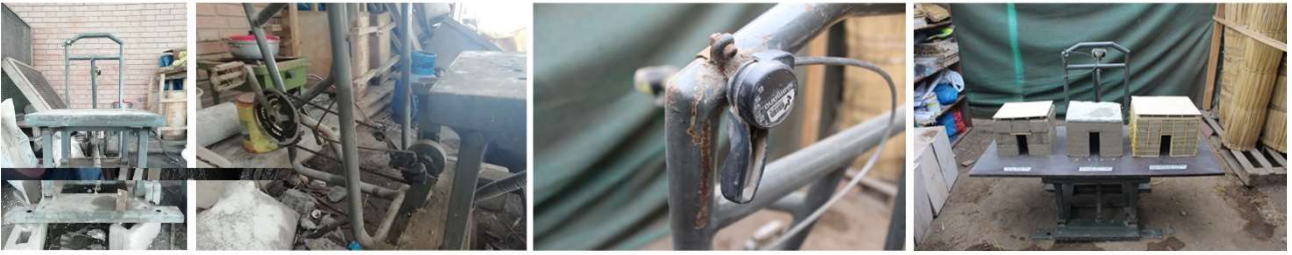
The construction of the unreinforced rammed earth prototype
