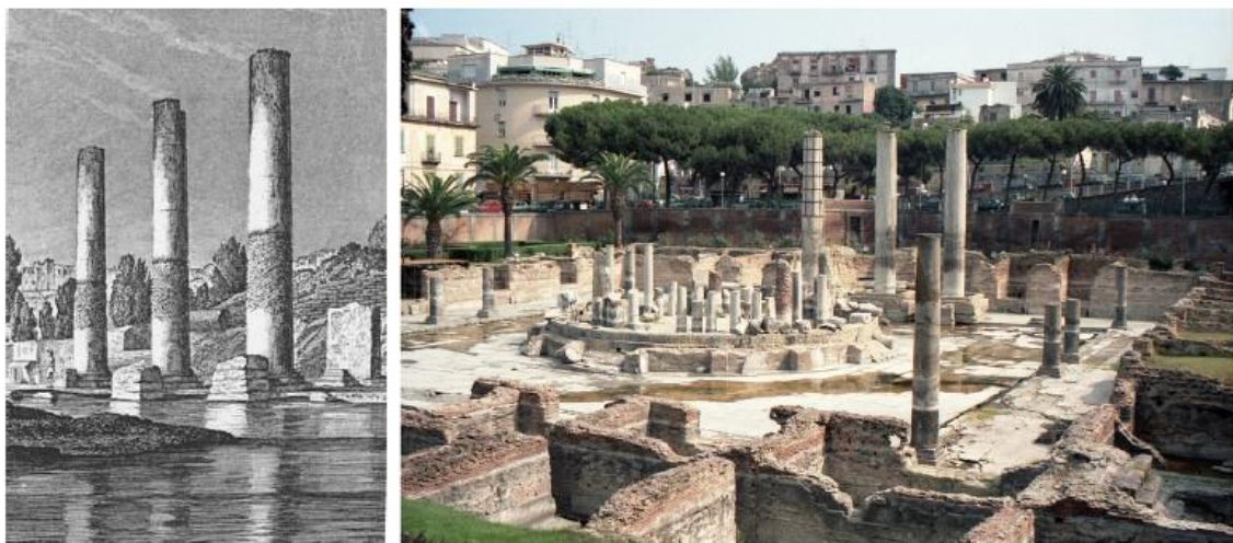
FIGURE 64.12 The ruins of the market of Serapeo at the center of Campi Flegrei caldera (Naples, Italy) provide a classic example of long-term caldera unrest. When built in ancient Roman times, the market must have been above sea level, yet by 1834 (left), it had sunk below sea level, and the mollusk borings more than a meter up the columns indicate lengthy periods even further below sea level prior to this. However, recent surveying measurements show that the region rose by 3.3 m between 1969 and 1984, raising the whole market well above sea level again by 1991 (right).
