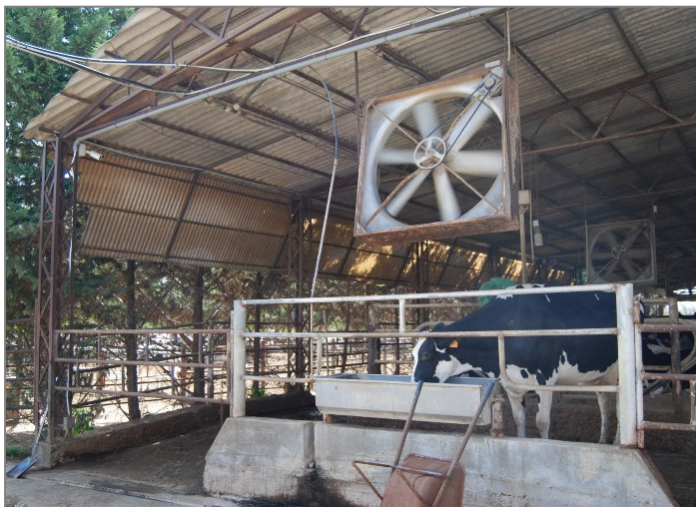
North-West front of the barn
