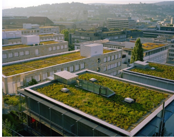
FIGURE 2.7: View of green roofs in Stuttgart, Germany [Internet]
