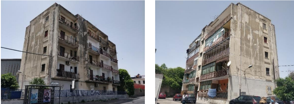
Figure 6.4. Multi-storey apartment building selected as case study 2.
