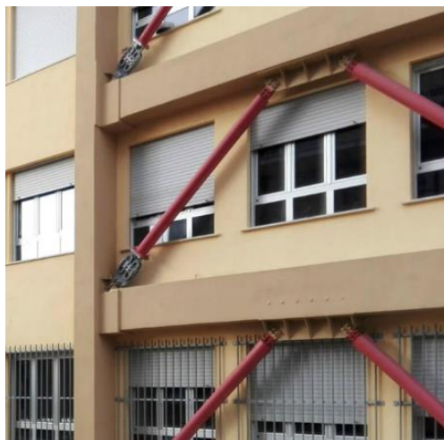
Figure 2.4. Addition of (a) steel buckling restrained brace (BRBs) and (b) hysteric dissipative steel brace
