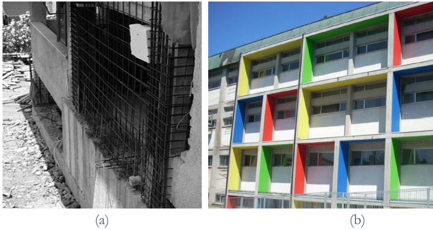
Figure 2.3. Addition of new RC shear walls (a) along the perimeter and (b) outside the existing building (image 2.3a from [11])
