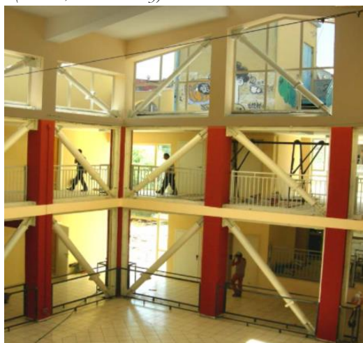
Figure 2.4. Addition of (a) steel buckling restrained brace (BRBs) and (b) hysteric dissipative steel brace
