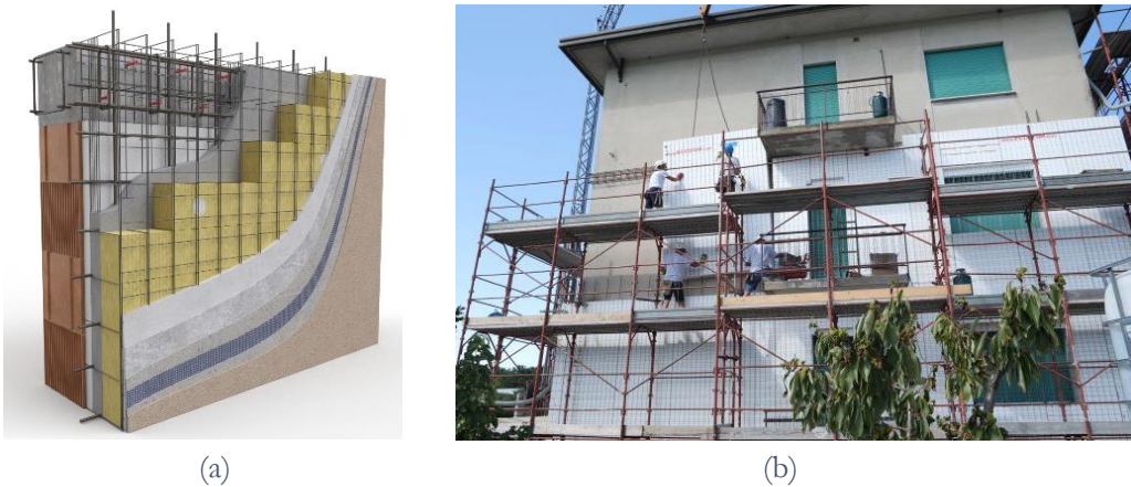
Figure 2.10. “Geniale cappotto sismico” system: (a) components and (b) application to a residential building located in Treviso (Northern Italy) [35]
