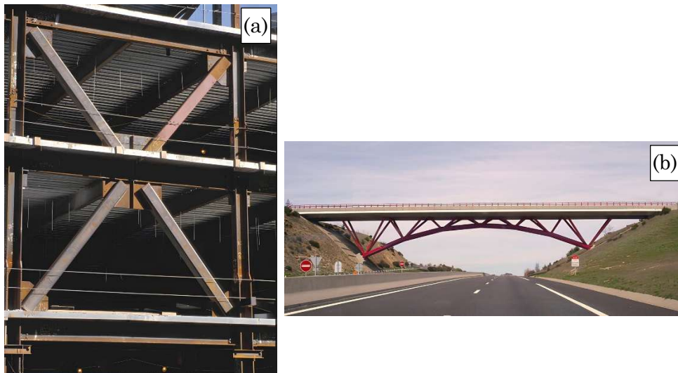
Fig. 4 – (a) HSS members used in braced structures [4]; (b) Composite road bridge, Marvejols, France [5].
