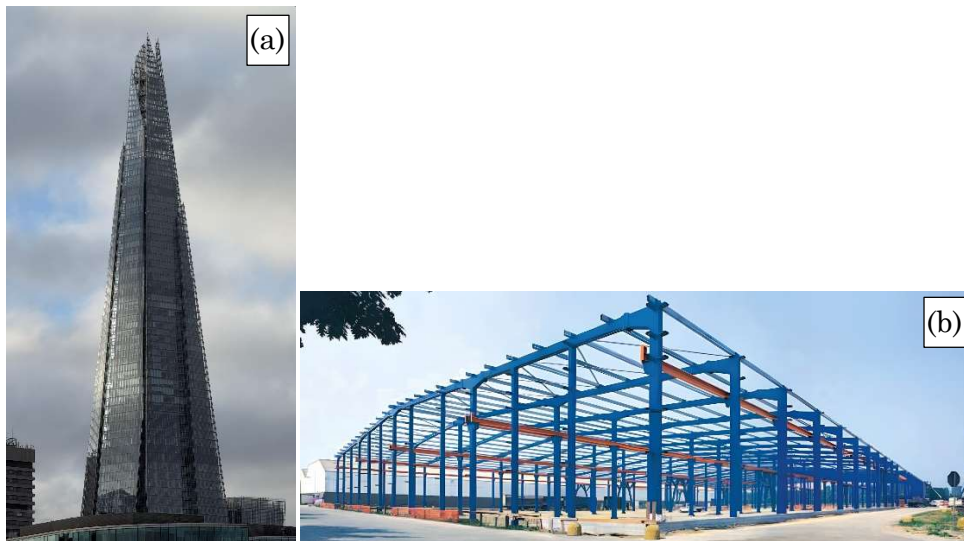
Fig. 3 – Examples of applications of hollow structural sections (HSS): (a) The Shard (London), employing hollow section steel members; (b) square HSS members in a steel moment-resisting frame [3].
