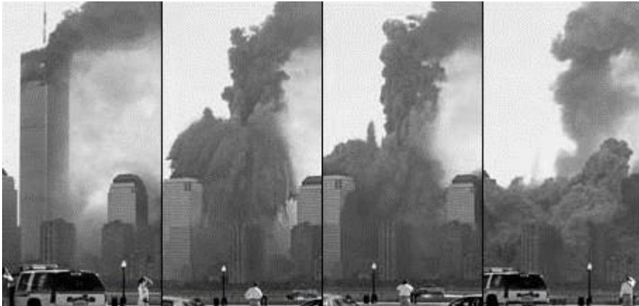
Figure 2.5 Collapse of the World Trade Center NY City [2001]
