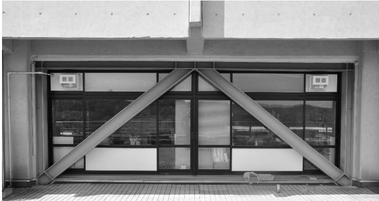
Figure 7.3 Steel Braced Frame
