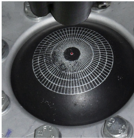
Fig. 19. Laser check of the bolts tightening.
