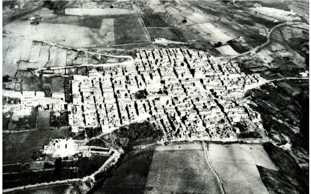
Figure 3. Aerial view of Poggioreale in the aftermath of the earthquake. Major effects are located in the lower part of the settlement close to the border of the urban fabric (courtesy of G. Coco).
