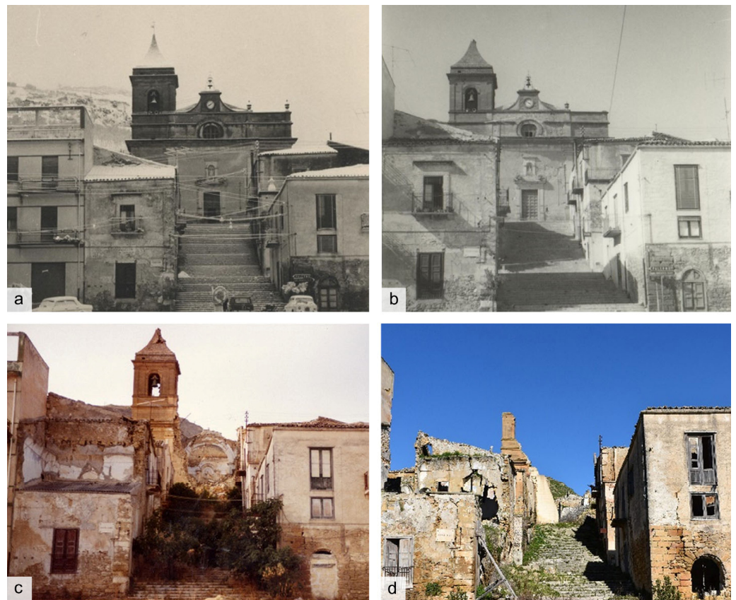
Figure 6. The main church of Poggioreale before and in the aftermath of the earthquake (a) and (b) (courtesy of G. Coco); in the early 2000s (c) (courtesy of G. Coco); and in 2022 (d) (authors' photo).
