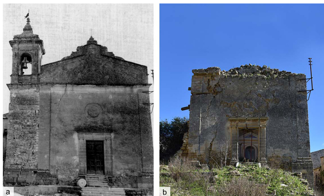
Figure 8. Gesù e Maria Church in the aftermath of the earthquake (a) (courtesy of G. Coco) and in 2022 (b) (authors' photo).
