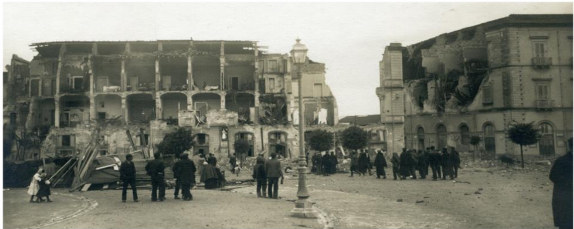
Figure 2 - Messina earthquakes (1908): OOP failures of external walls [17]
