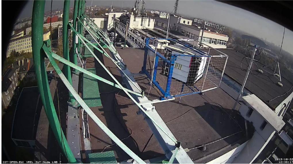
Figure 10.4: VREL SUT roof top thermal smart house laboratory End Node ( [125] ).
