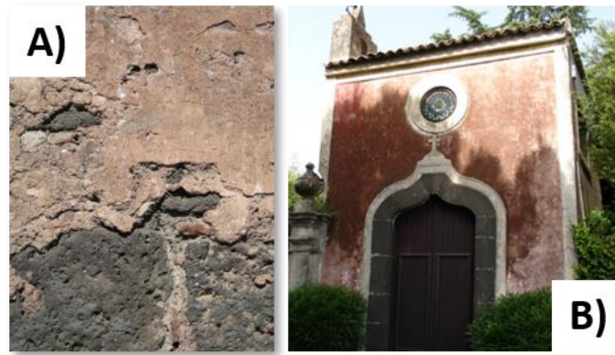
Fig. 1.13 – Example of ancient applications: a) Detachment of historical mortar based on ghiara; b) Original plaster application in San Salvatore church in Viagrande, Catania, Italy.
