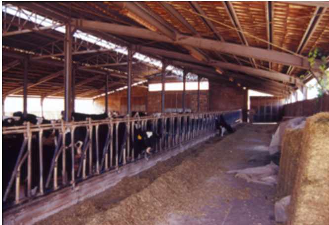
Figure 2 - Barns roof system realized with wooden supporting structures and roofing tiles
