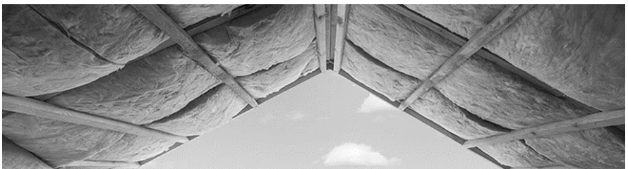
Figure 3 - Example of sheep wool insulations on roof
