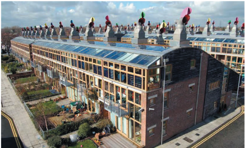
Figure 19. BedZED (Source: Tom Chance., 2007).
