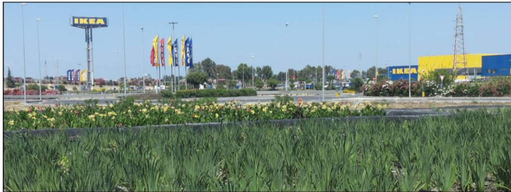
Figure 3.4: CWs hybrid system at the IKEA store in Catania
