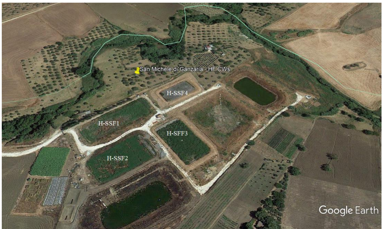
Figure 3.7: Satellite map of CW system at San Michele di Ganzaria plant (Eastern Sicily)
