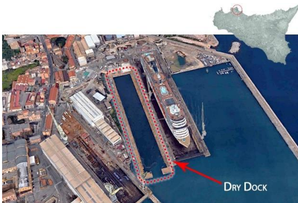
Figure 7-18: Top view of the Dry Dock subject to intervention within the Palermo Industrial Port.
