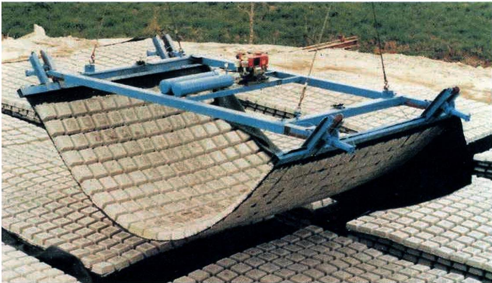
Figure 7-30: Prefabricated Trevimat modules.
