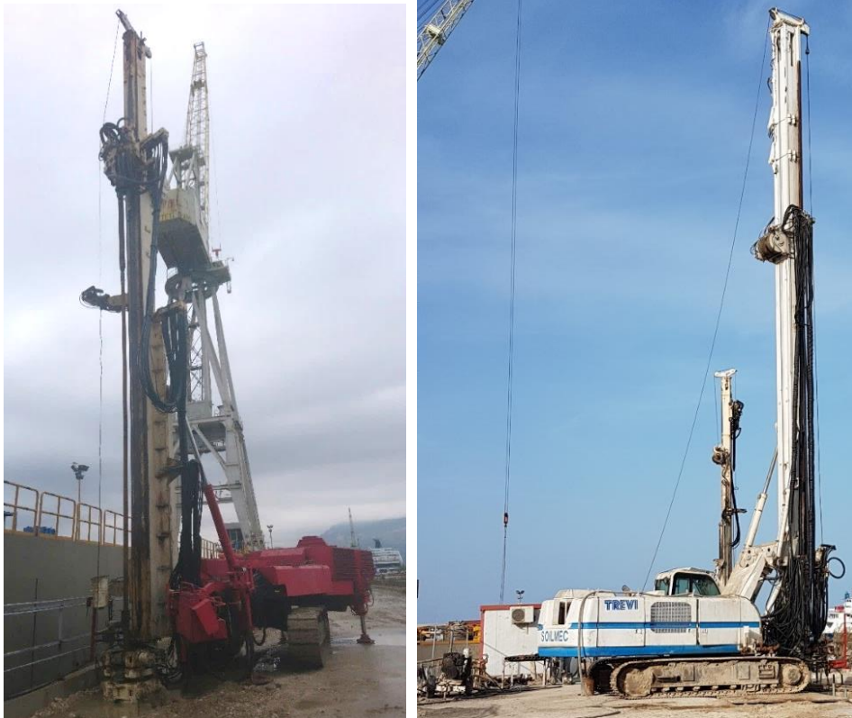
Figure 7-20: Some of the microdrilling used in the building site of Palermo.
