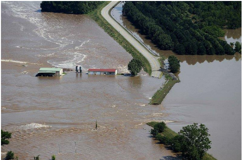
Figure 2-1: Flood waters from the Arkansas River rush through a broken levee 1 st June 2019 [Thomas Metthe - Arkansas Democrat Gazette 31st May 2019].
