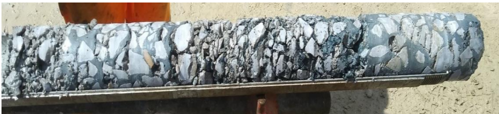
Figure 7-27: core drilling to evaluate the cement mixture performances.
