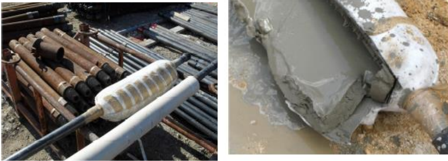
Figure 7-23: Shutter Bags after being pumping.
