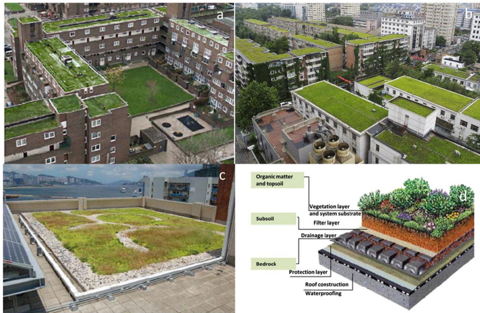
Figure 2.7. Extensive green roof: (a) Castleton et al., 2010; (b-c) Sam and Hui, 2009; (d) Stratigraphy ( http://www.zinco-greenroof.com/EN/downloads/pdfs/ZinCo_Intensive_Green_Roofs.pdf ).
