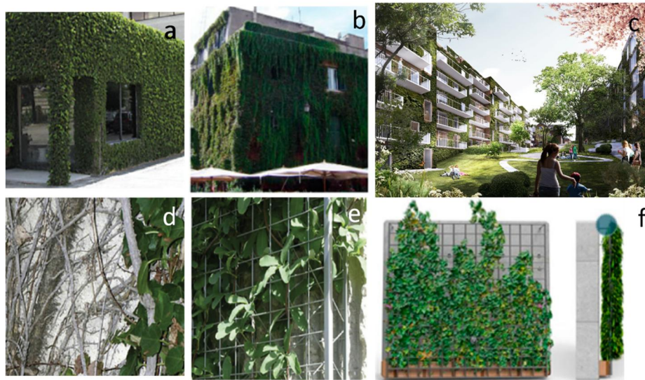
Figure 2.8. Green facades and support structures: (a-d) Typical green walls with self-clinging climbing plants (Kontoleon et al., 2010); (b-f) Green facades with modular trellis panel systems (Perez, et al. 2014).
