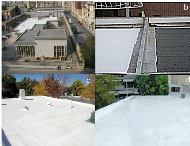
Figure 2.6. Building roofs coated with reflective paint: (a) Romeo, 2012; (b-c) Bozonnet et al., 2011; (d) Synnefa et al., 2012.
