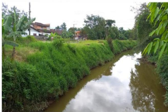
Figure 3 - Limited access to drainage pipelines due to vegetation along the riverbank
