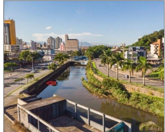
Figure 9 - Image of the Cachoeira River in Joinville-SC (Brazil) during low tide, showing drainage pipelines not submerged
