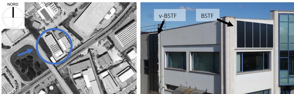
Figure 4.12 – Map of the building (left side), photo of the two BSTF prototypes (right side).
