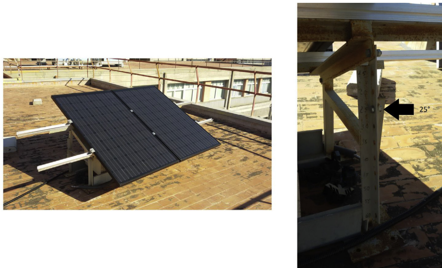
Fig. 1. Mounting structure: a) PV/T modules – b) Tilt angle setting structure, \beta .
