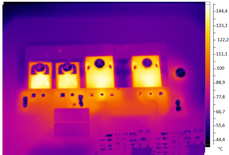
Figure 4.5: Thermal image of the phase switching cell
