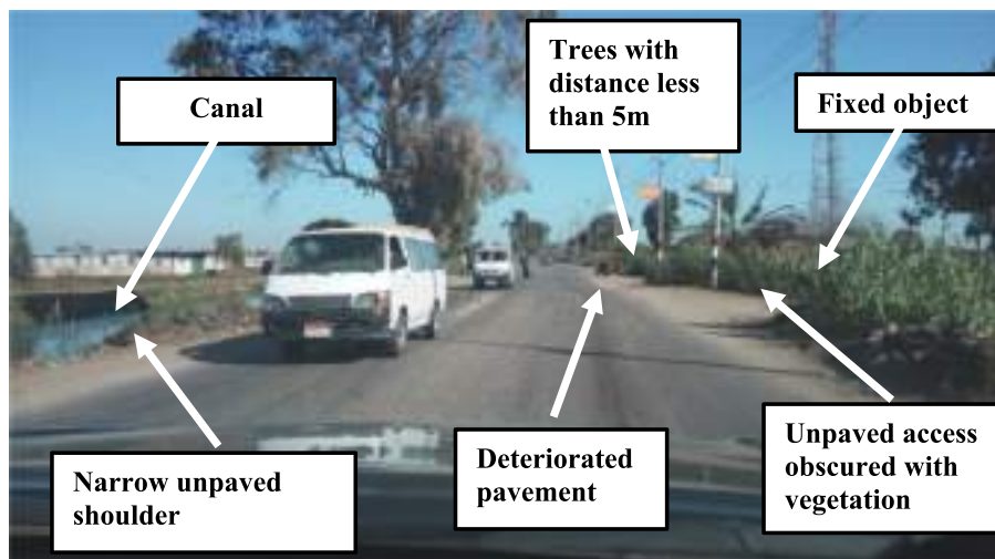
Fig. 5. Road Section Safety Issues.
