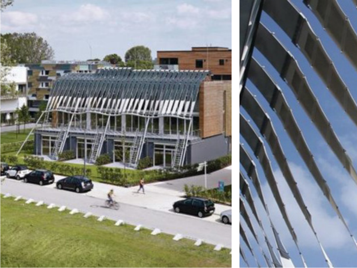
Fig. 2.13. Soft House, Amburgo (Kuipers and Engineering, 2015)
