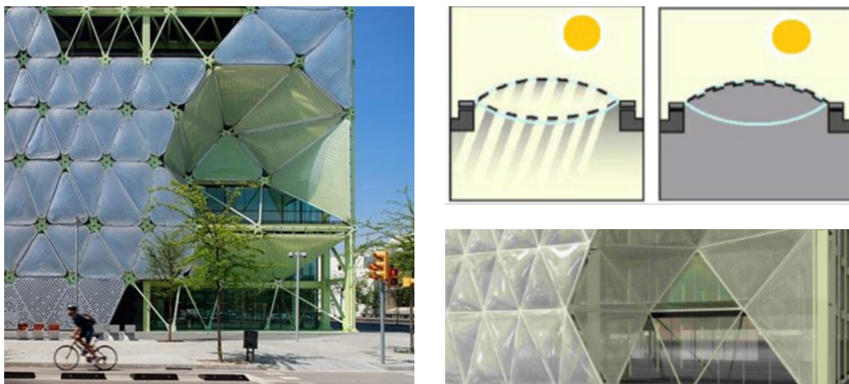
Fig. 2.4. Media-ICT building, Barcelona. (Shahin, 2019)
