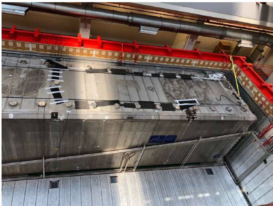
Figure 42. Picture taken after the positioning of the first cold vessel showing also the cold shields inlet pipes.
