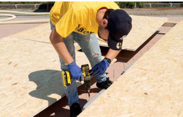
Figure 186/ Fixing of OSB boards - On-site - University Campus, Catania (CT)
