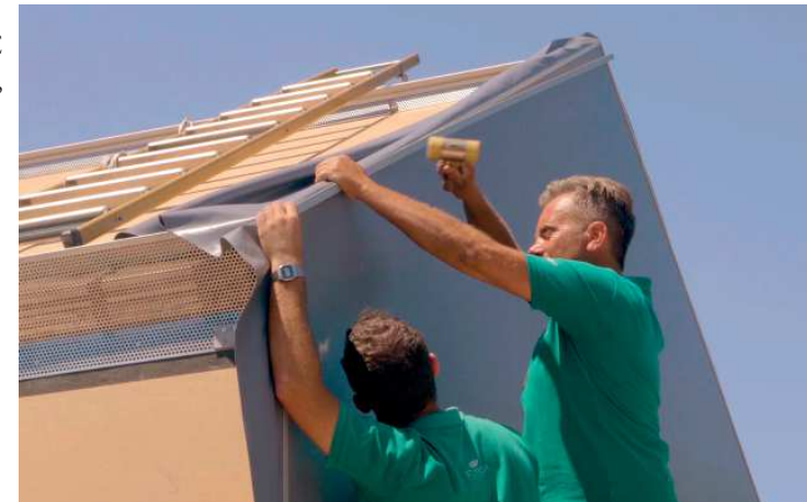
Figure 202 / Installation of the PVC textile - On-site - University Campus, Catania (CT)
