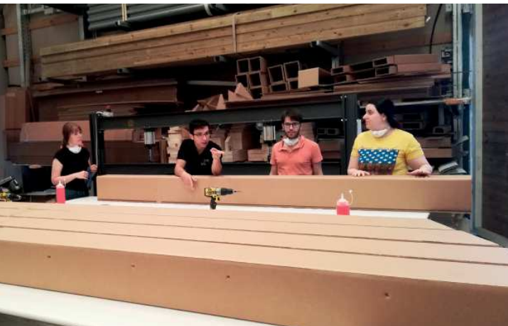
Figure 179 / Production of PACO 120 h380 cm - Off-site - Archicart Area srl, Giarre (CT)
