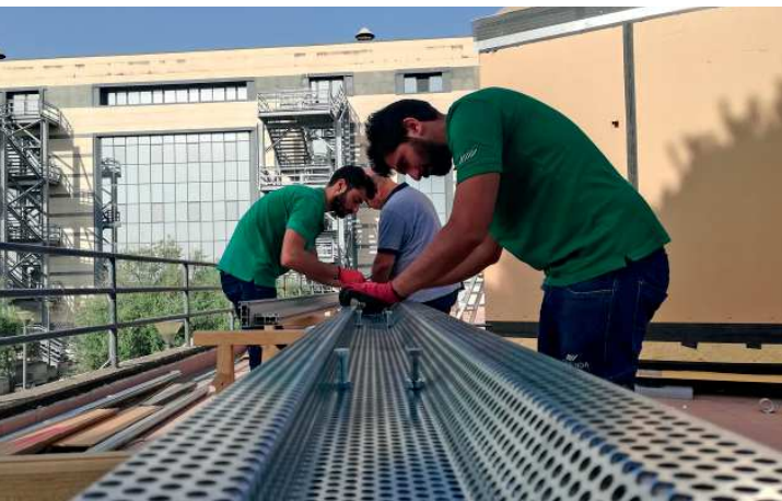
Figure 200 / Preparation of the holed galvanized folded steel sheet - On-site - University Campus, Catania (CT)
