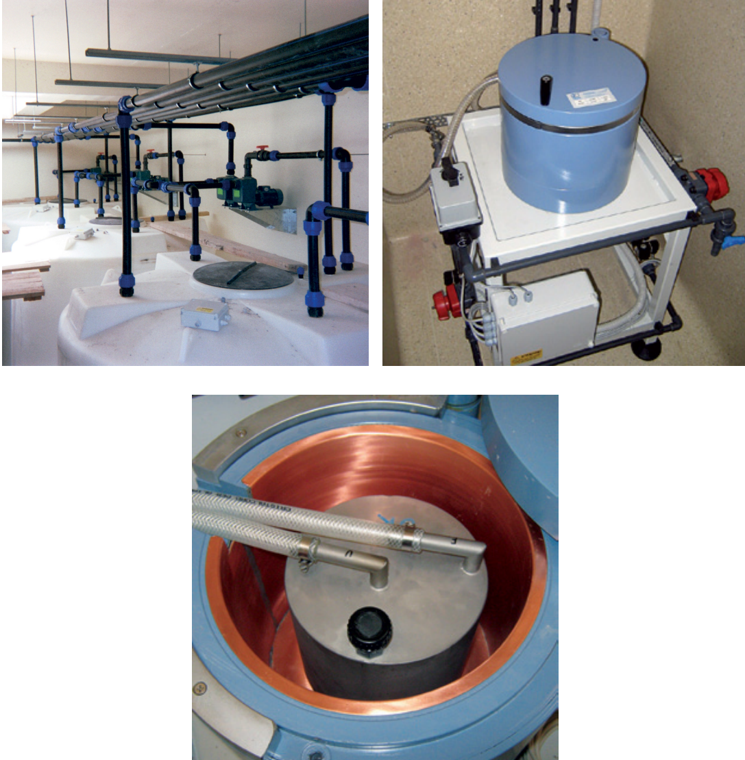
Figure 2.3: Installation of waste management system for liquid radioactive waste monitoring.
