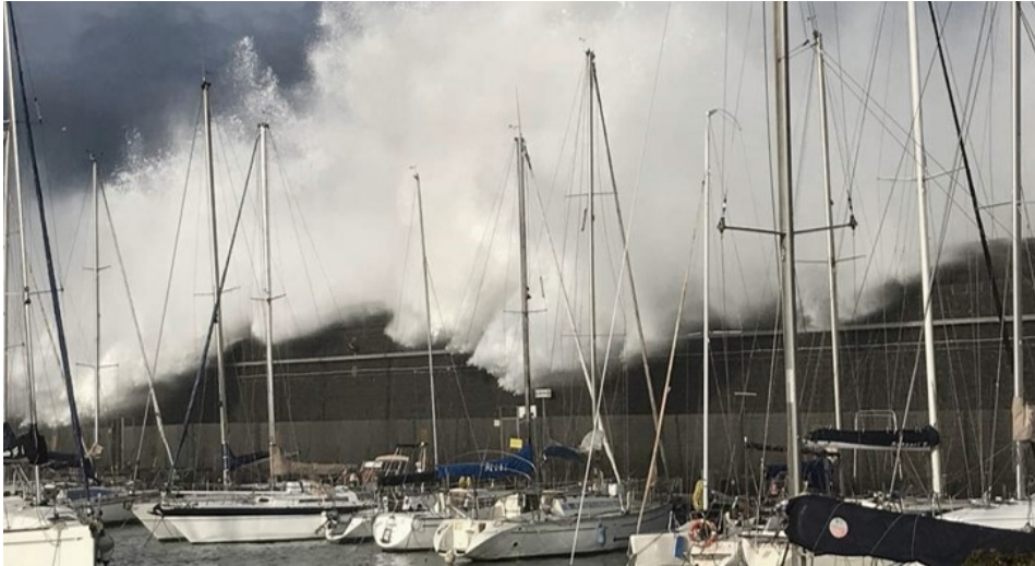
FIGURE 3.4 Overtopping discharge over the Catania harbor breakwater caused by the extreme marine event occurred in February 2019. Source: newspaper La Sicilia of 5th July 2021.
