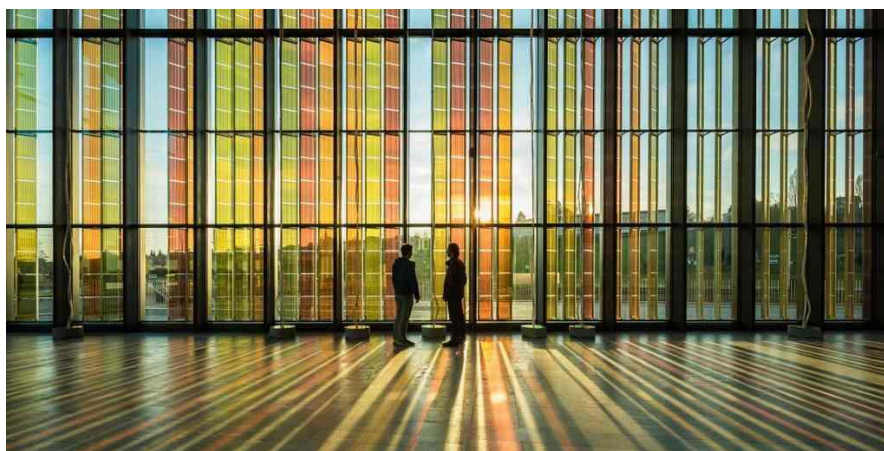
Figure 1.25. Dye solar cell façade at SwissTech convention center at EPFL, by Solaronix.
