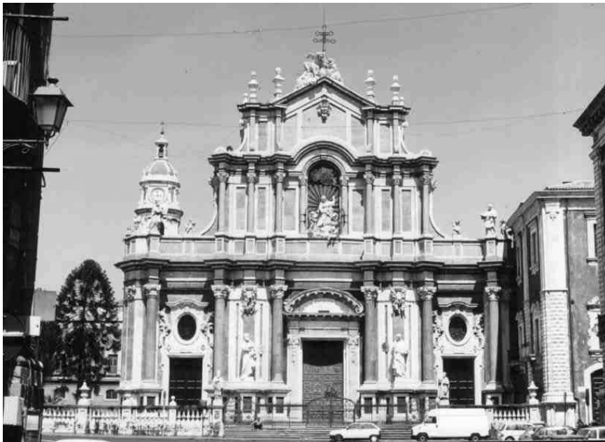
Figure 5: Main prospect of the Cathedral.
