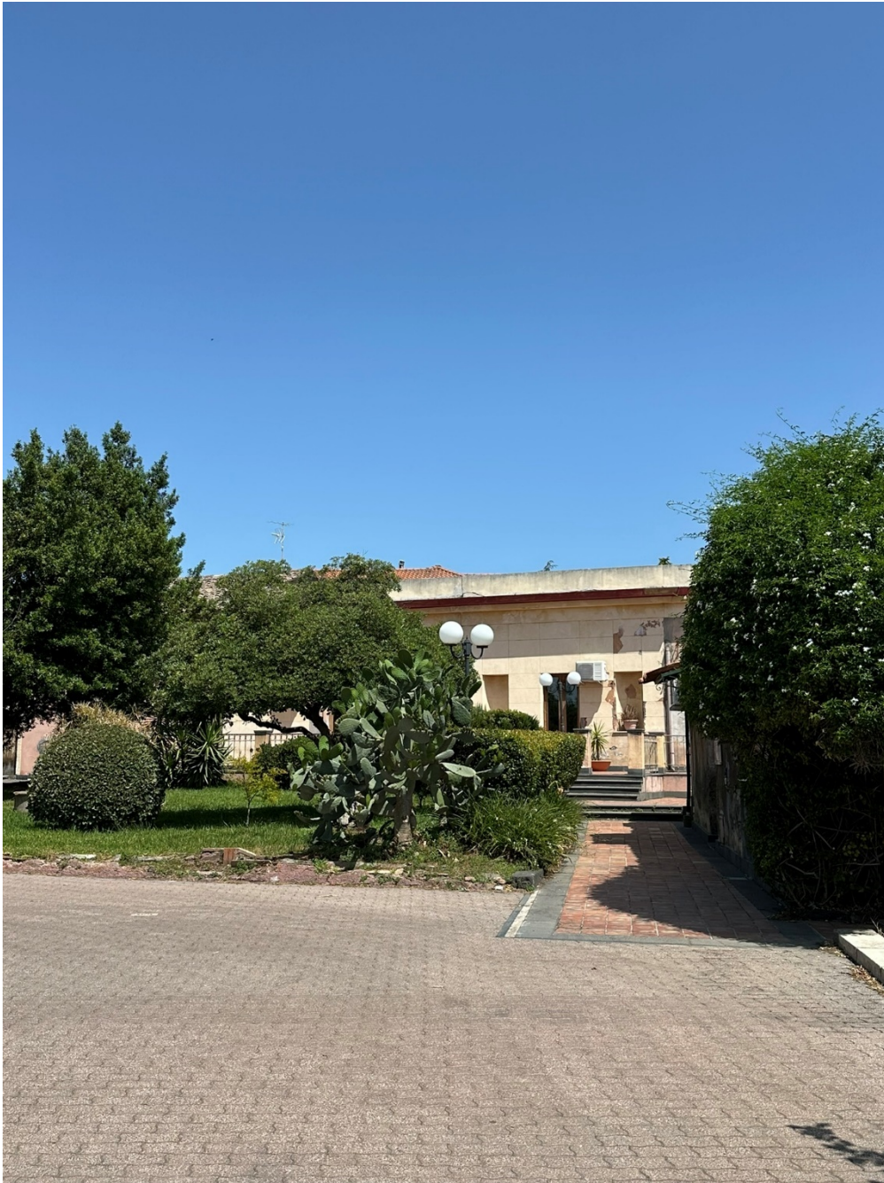
Figure 108_External photo of the building surveyed of Delegazione Comunale located in Via del Bosco, 19
