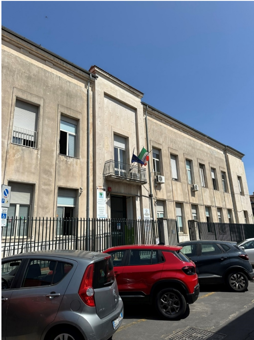
Figure 45_External photo of the building surveyed of ICS Fava complex located in Via Timparello, 53
