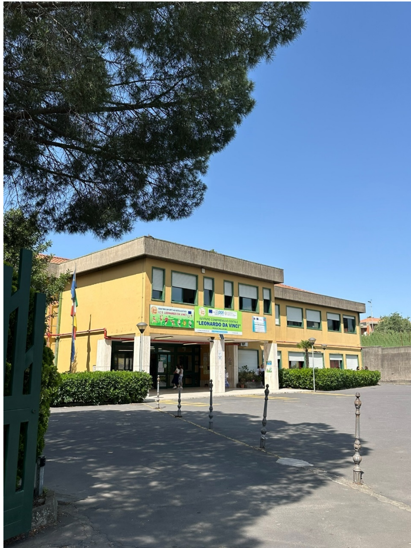
Figure 79_ External photo of the building surveyed of ICS Leonardo Da Vinci complex located Via della Regione Siciliana, 12
