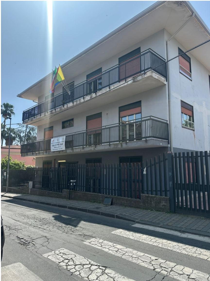
Figure 37_ External photo of the building surveyed_ Via dei Villini, 19
