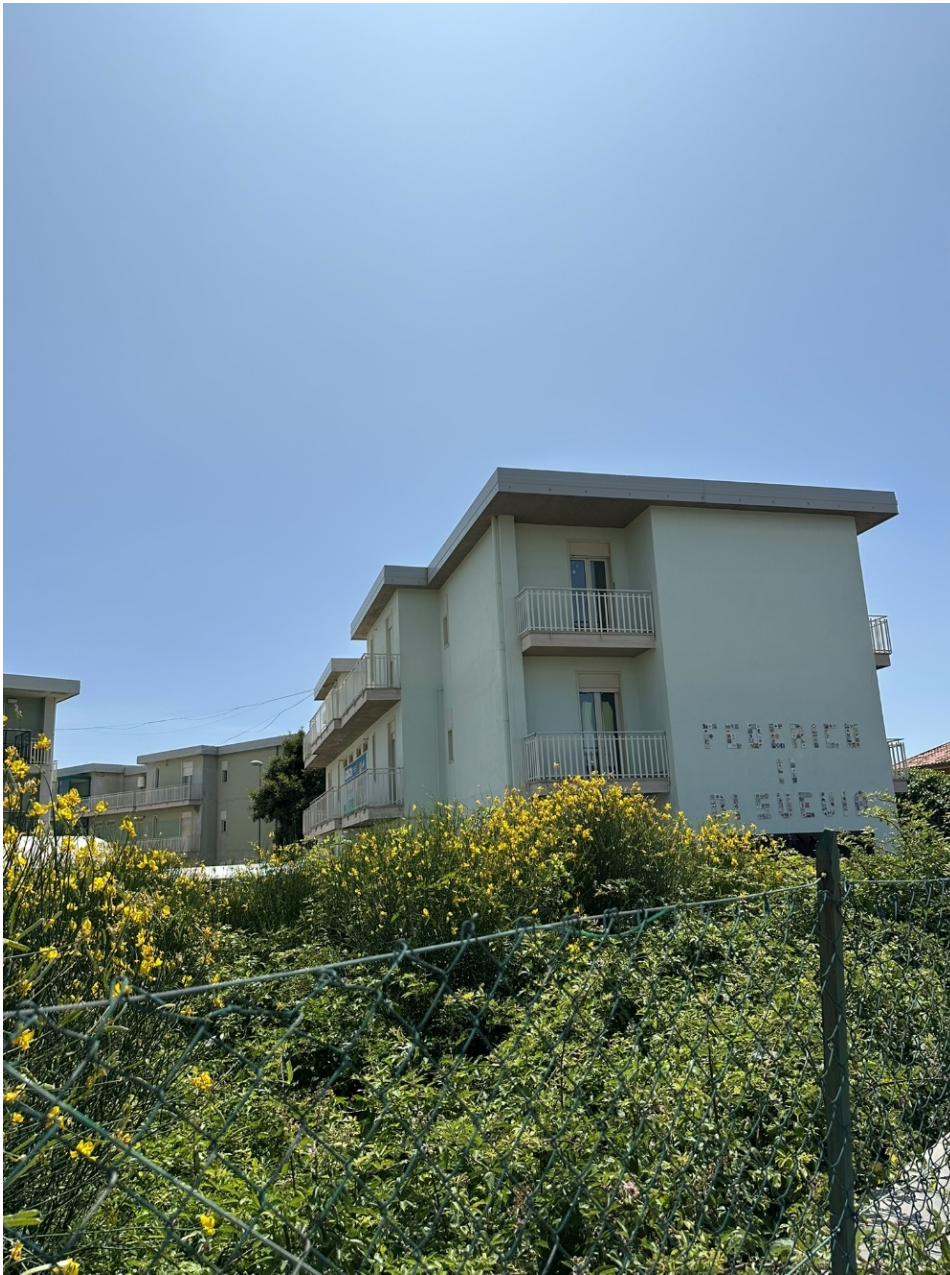
Figure 58_External photo of the building surveyed of ICS Federico II complex located in Via Massimo D’Azeglio, 14
