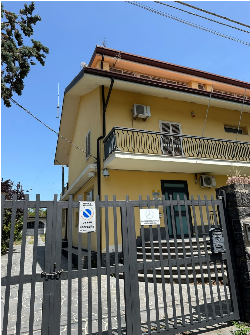
Figure 102_External photo of the building surveyed of Ufficio Protezione civile located in Via Manzoni, 8
