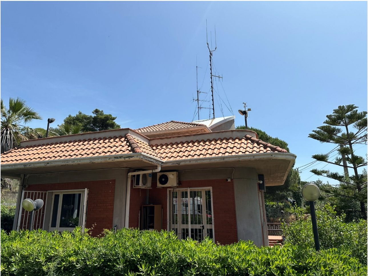
Figure 114_External photo of the building surveyed of Croce Rossa Italiana located in Via Petrarca, 24
