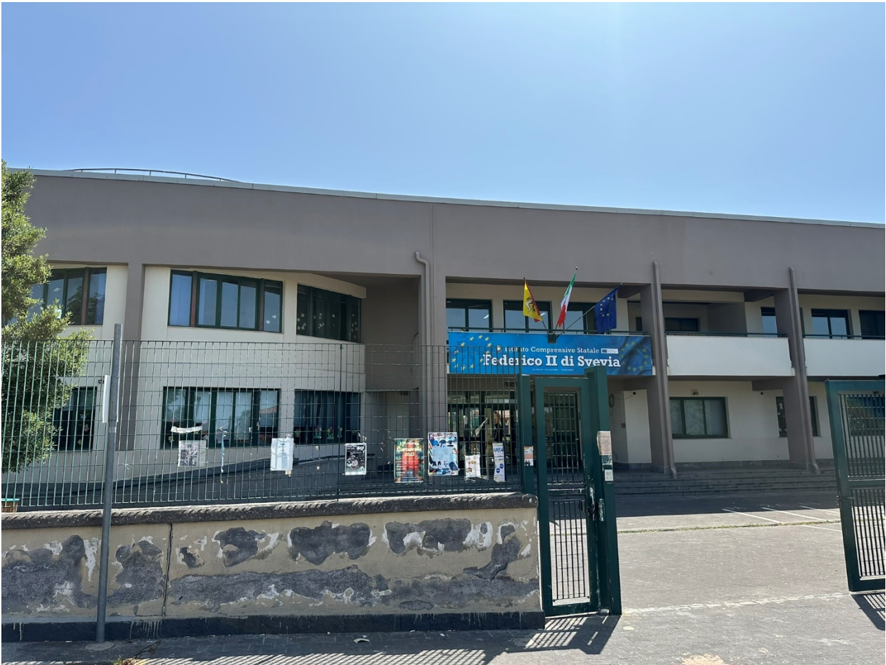
Figure 65_ External photo of the building surveyed of ICS Federico II complex located Via del Sole,2
