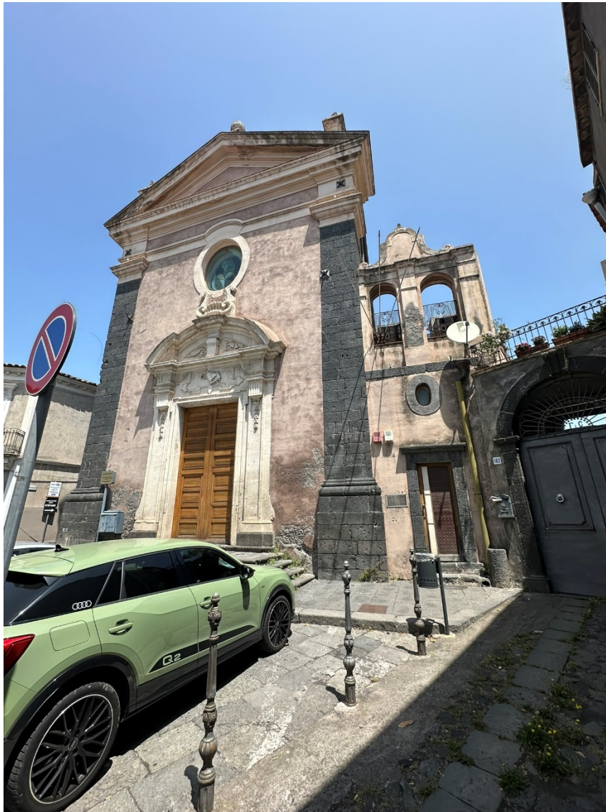
Figure 122_External photo of the building surveyed of Auditorium located in Via San Nicolò
