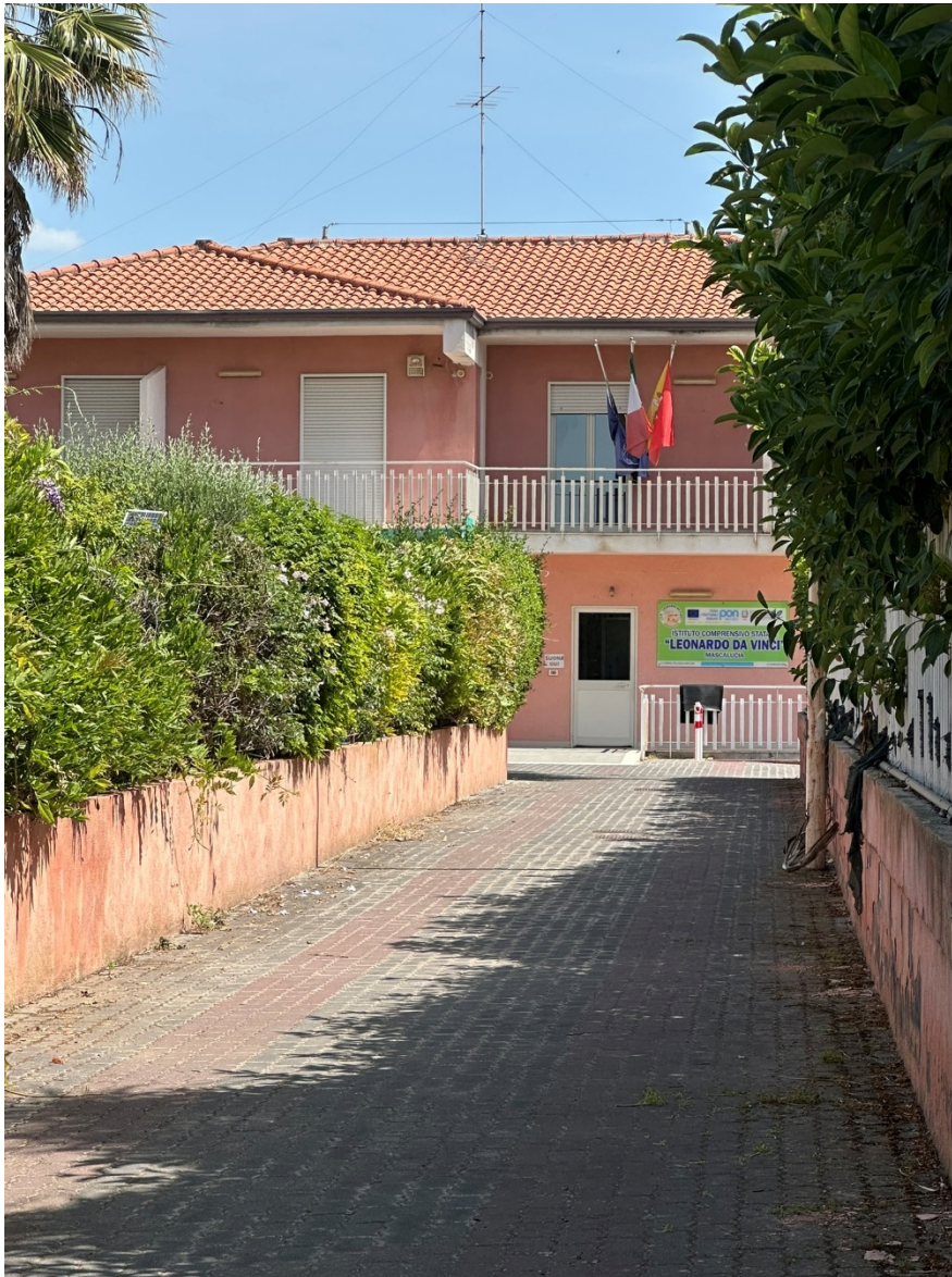
Figure 71_ External photo of the building surveyed of ICS Leonardo Da Vinci complex located Via Roma, 217
