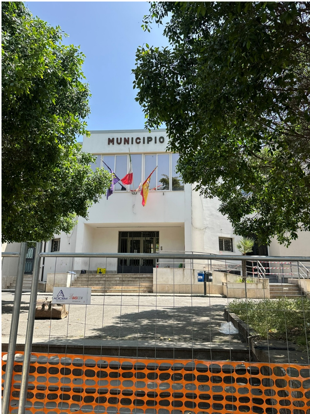
Figure 96_External photo of the building surveyed of Municipio located in Corso San Vito, 2
