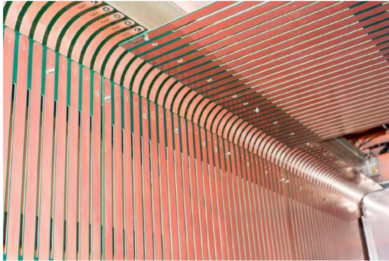
Figure 4.8: A corner of the 35-t TPC field cage during construction
