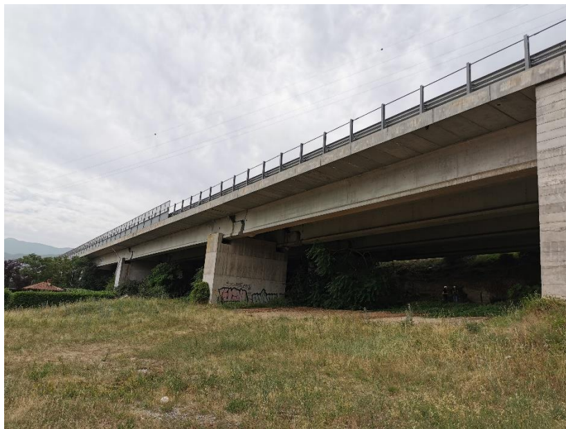
Fig. 4.1. Picture of the Avezzano viaduct
