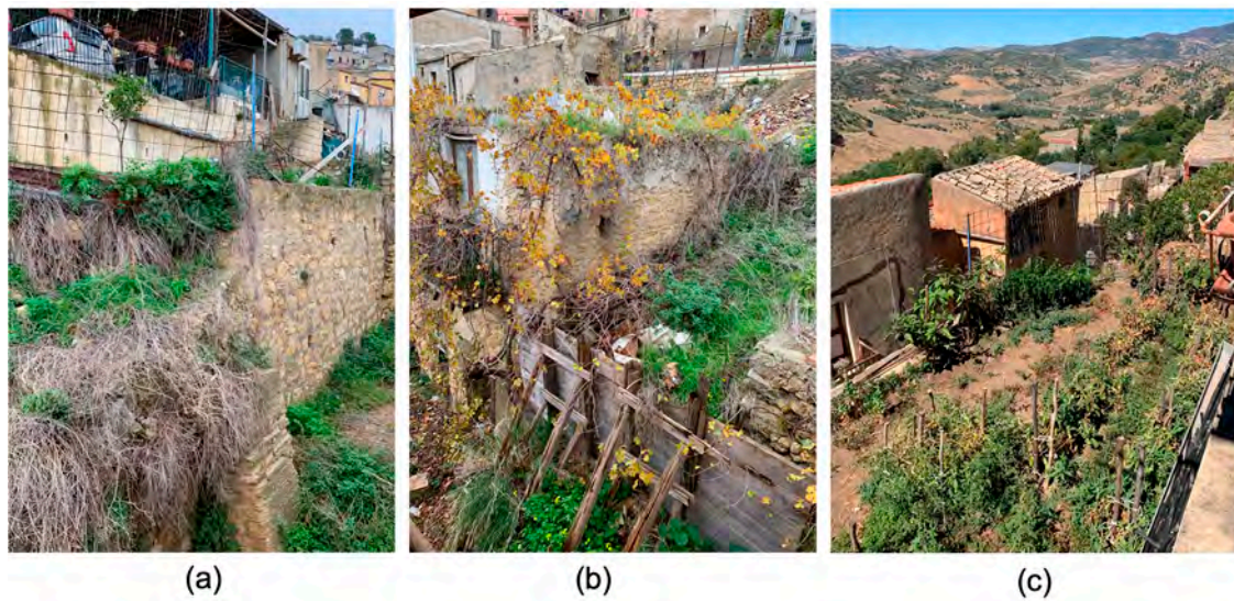
Figure 8. Partial demolition and securing along and between vico Vitale and via Riscato. (a,b) The downstream situation shows the provisional shoring and partial reconstruction of the retaining wall. (c) Upstream situation with the use of the infilled area as a private vegetable garden.
