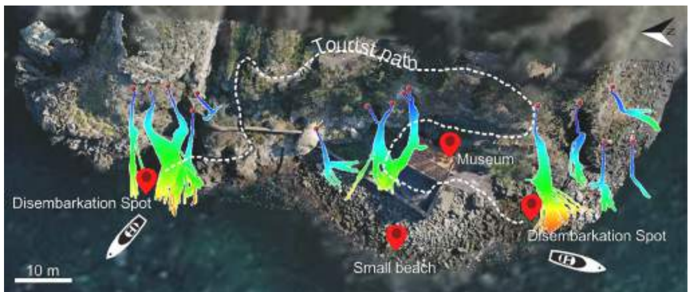
Fig. 8. Impact scenario of rockfall hazard on the main elements at risk.
