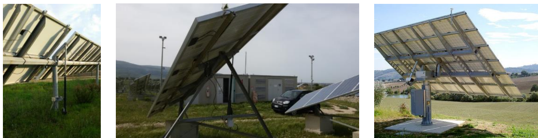
Figure 6. Left: example of single-axis tracker, tilt 0^\circ . Center: example of single-axis tracker, tilt 20^\circ . Right: example of dual-axis tracker
