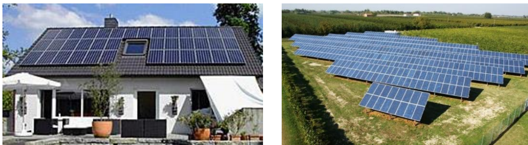
Figure 7. Left: example of rooftop PV plant. Right: example of ground-mounted PV field
