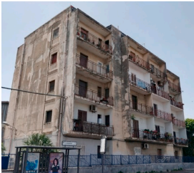
Fig. 4. The pilot building in its current state.
