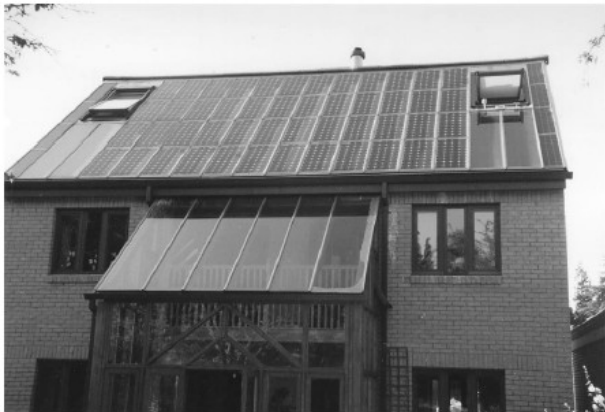
Figure 22 PV roof installation
