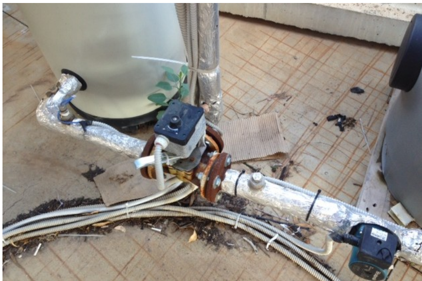
Figure 3. The 3-way mixing valve.
