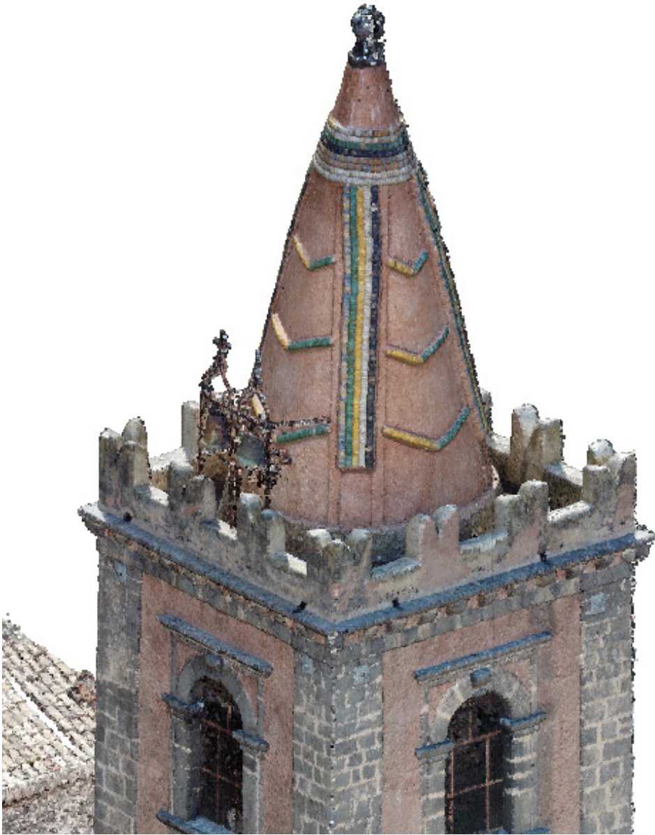
Figure 114. Detail of the photogrammetric point cloud of the spire of San Pietro.
