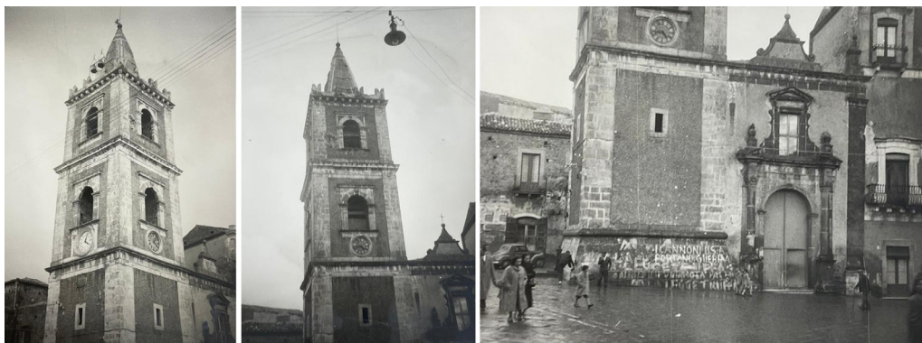
Figure 104. Photographs of February 1955 of the Church of San Pietro. Source: Photographic archive of the Soprintendenza per i Beni Culturali e Ambientali di Catania, CT 6-19, photos n. 6393, 6394, 6392.
