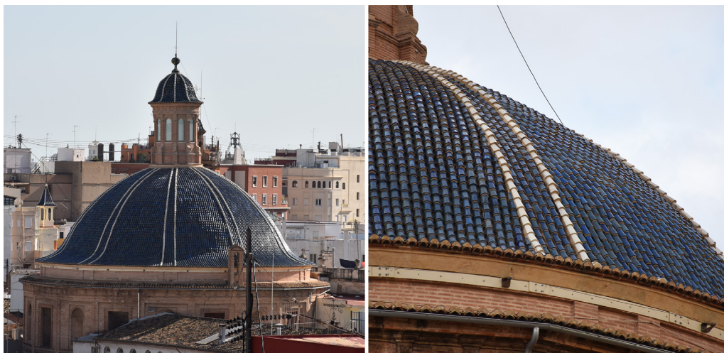
Figure 127. Detail of the ceramic tile cladding of the Escuelas Pías dome.
