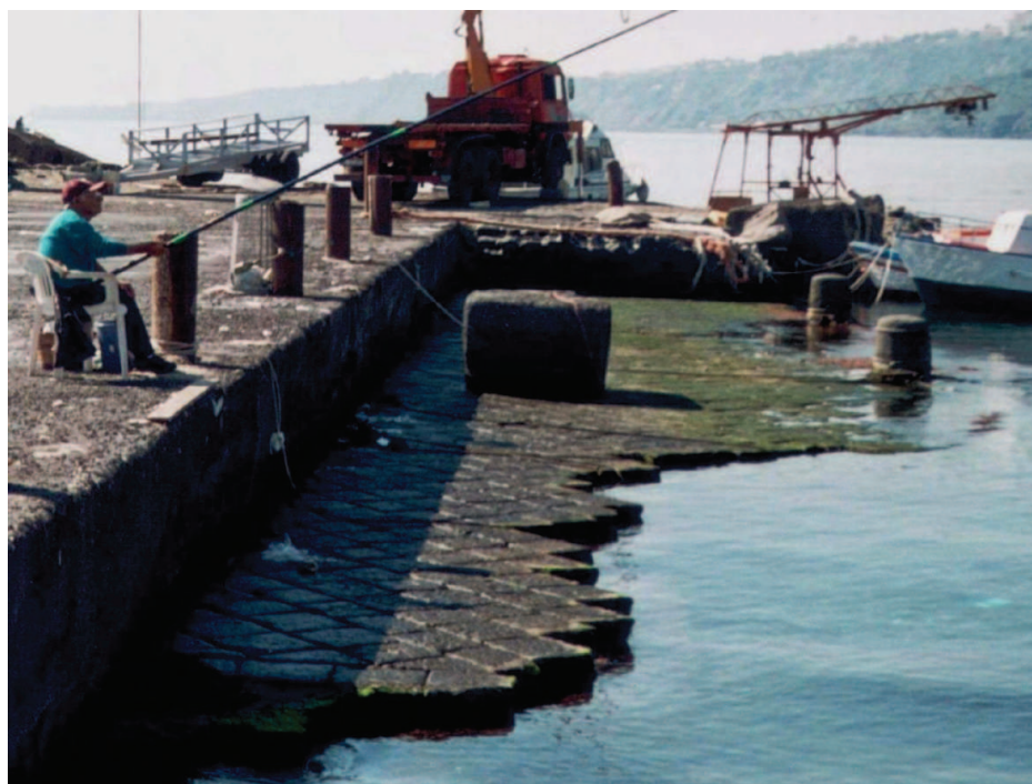
Fig. 6. Old and new docks in the Stazzo port during ebb tide.
