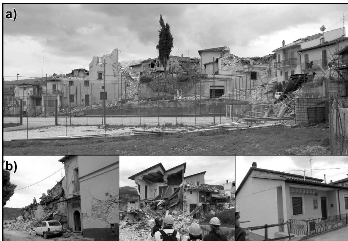
Fig. 3 - Onna: a) view of the village with several collapsed houses; b) inside the village, different damage grades depending on building typology.
