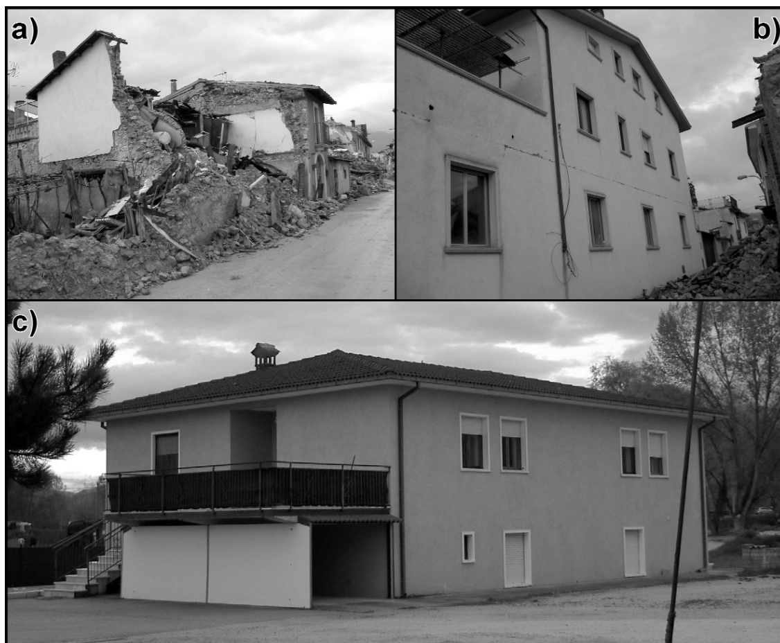
Fig. 5 - Onna, examples of damaged buildings with different vulnerability: a) class A, total collapse (grade 5); b) class C, slight damage (grade 2); c) class D, undamaged.
