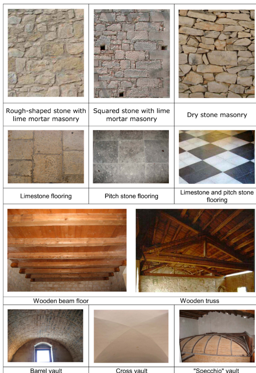
Figure 2. Materials and building techniques common to Donnafugata Castle and TRBs in its surrounding area.
