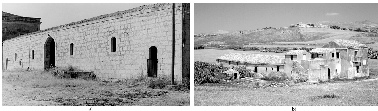
Figure 1. Examples of traditional rural masonry buildings located in Eastern Sicily.
