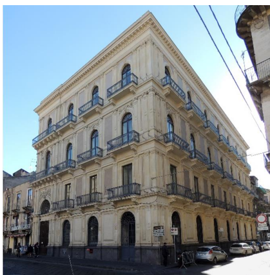
Figure 1. North- and west-facing façades of the selected building.
