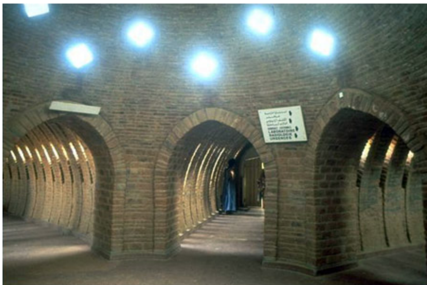
Central Market Rehabilitation, Mopti, Mali
