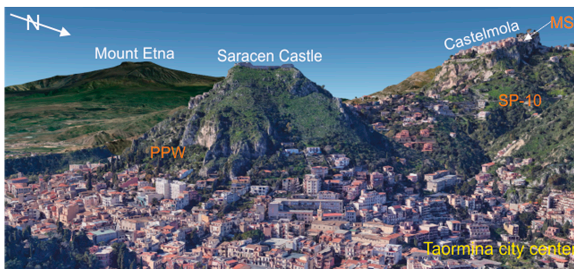
Figure 2. Location of the most relevant spots threatened by rockfall in the Taormina complex. Key: PPW—pedestrian pathway; SP-10—Provincial Road 10; MS—Castelmola Main Square.
