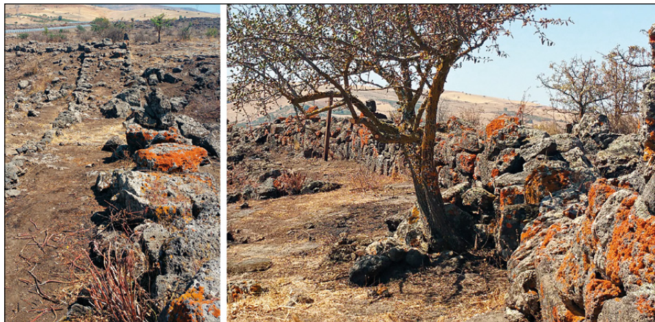
Fig. 8 – Wall structure (survey of 31-Aug-2017) visible after a terrible fire (photo by the authors).
