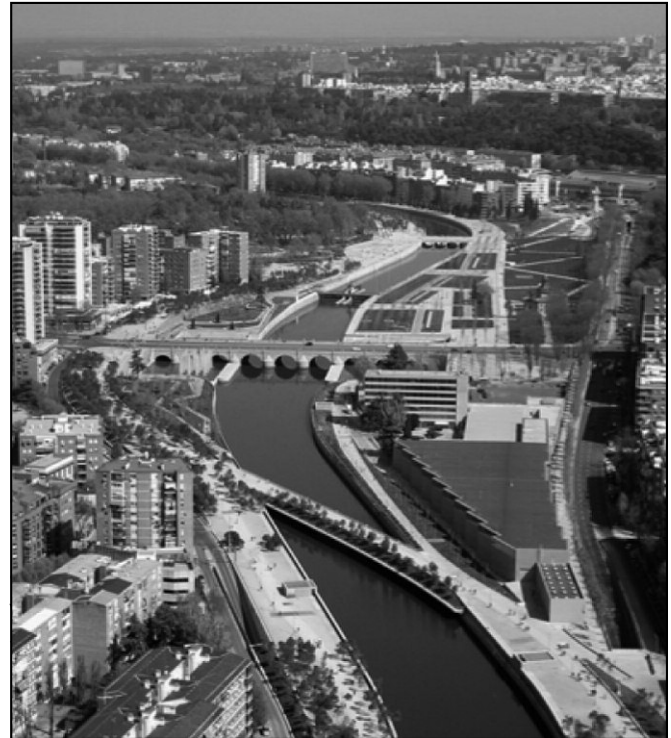
Figure 2 - View of the Manzanares River
