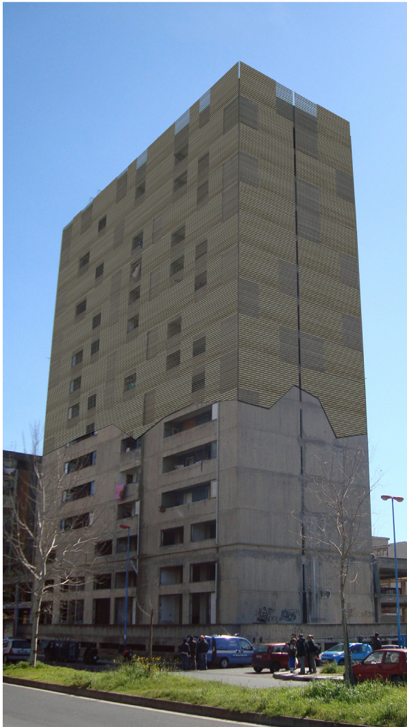
Figure 4: The “Concrete building” in Catania: current façade (lower part) and simulation of the new solar thermal coating (upper part).
