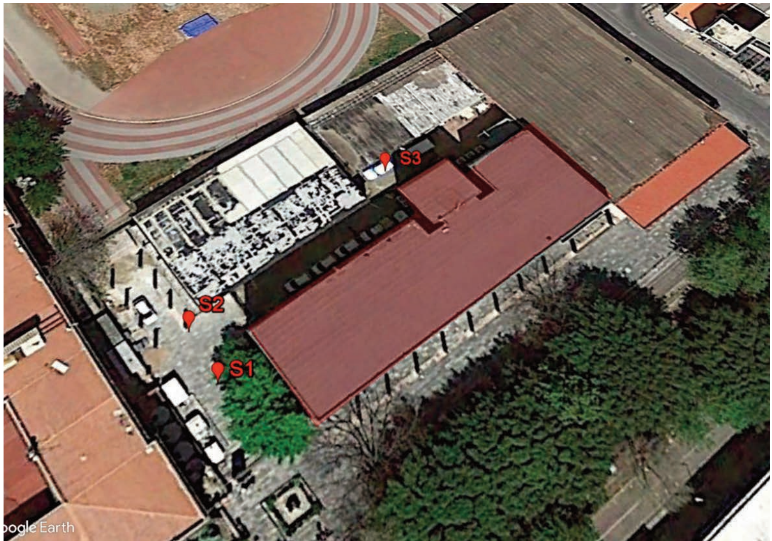
FIGURE 3. Layout of the test site with boreholes location in the “Civil Defence Department” (DPC) area.
