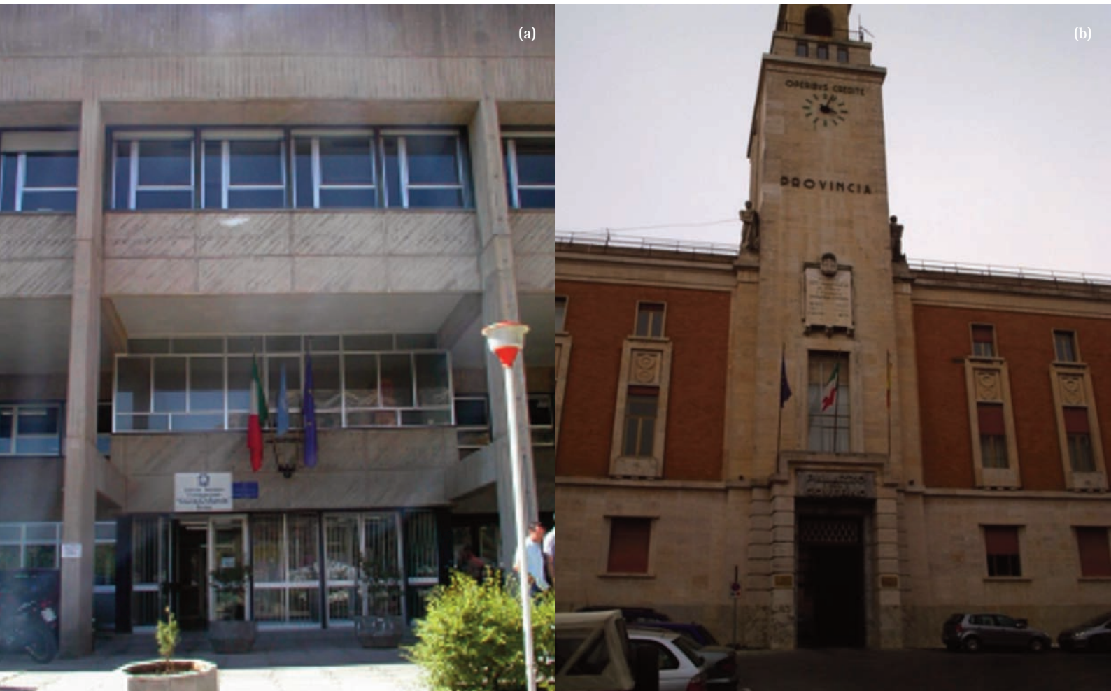
FIGURE 2. Reinforced concrete building: Duca D'Aosta School (a); masonry building: Palace of the Regional Province of Enna (b).
